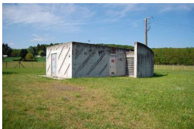
Station de pompage de Gresswiller
